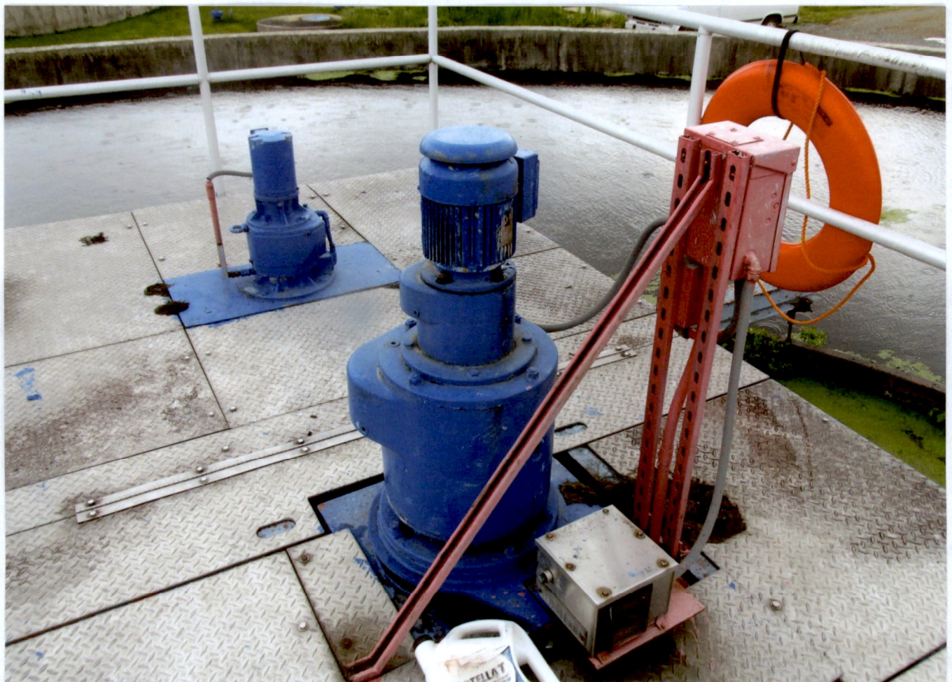
9, NORTH CLARIFIER- DOWN FOR GEAR DRIVE REPAIR
