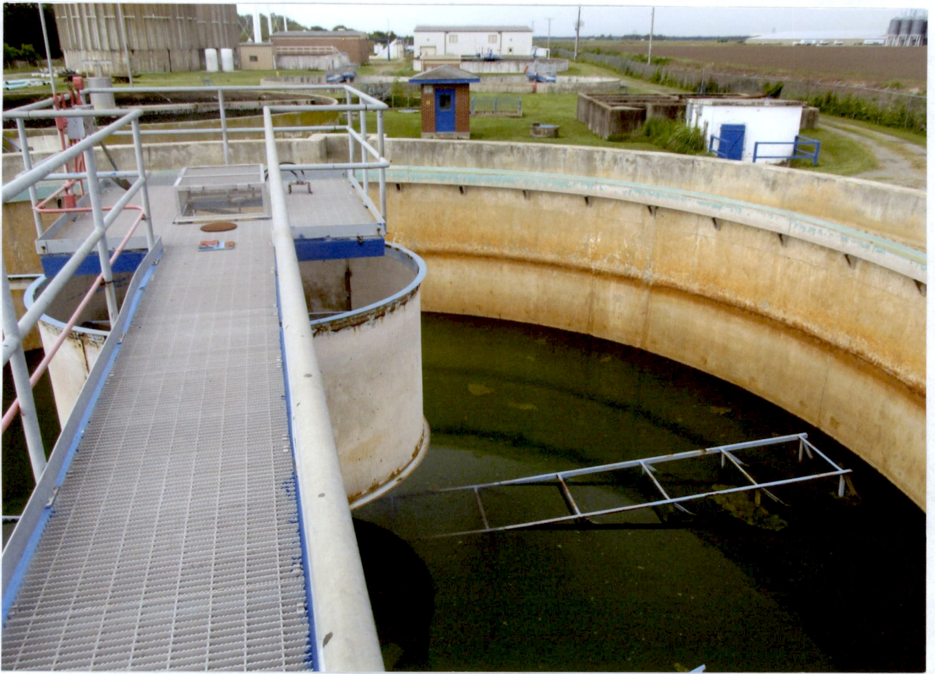
4. LARGER PRIMARY CLARIFIER - GEAR DRIVE OUT FOR REPAIRS
