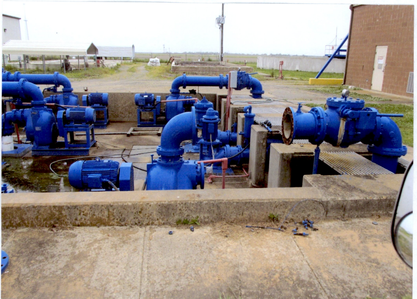
8. BIO TOWERS RECIRCULATION PUMP STATION - REPAIRS MADE BACK IN SERVICE
