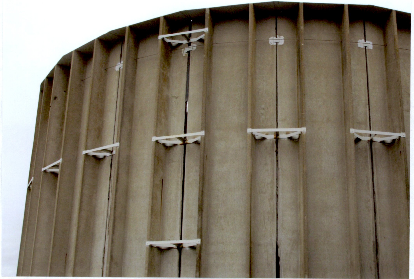
7. BIO TOWER FIELD REPAIRS TO STRUCTURE
