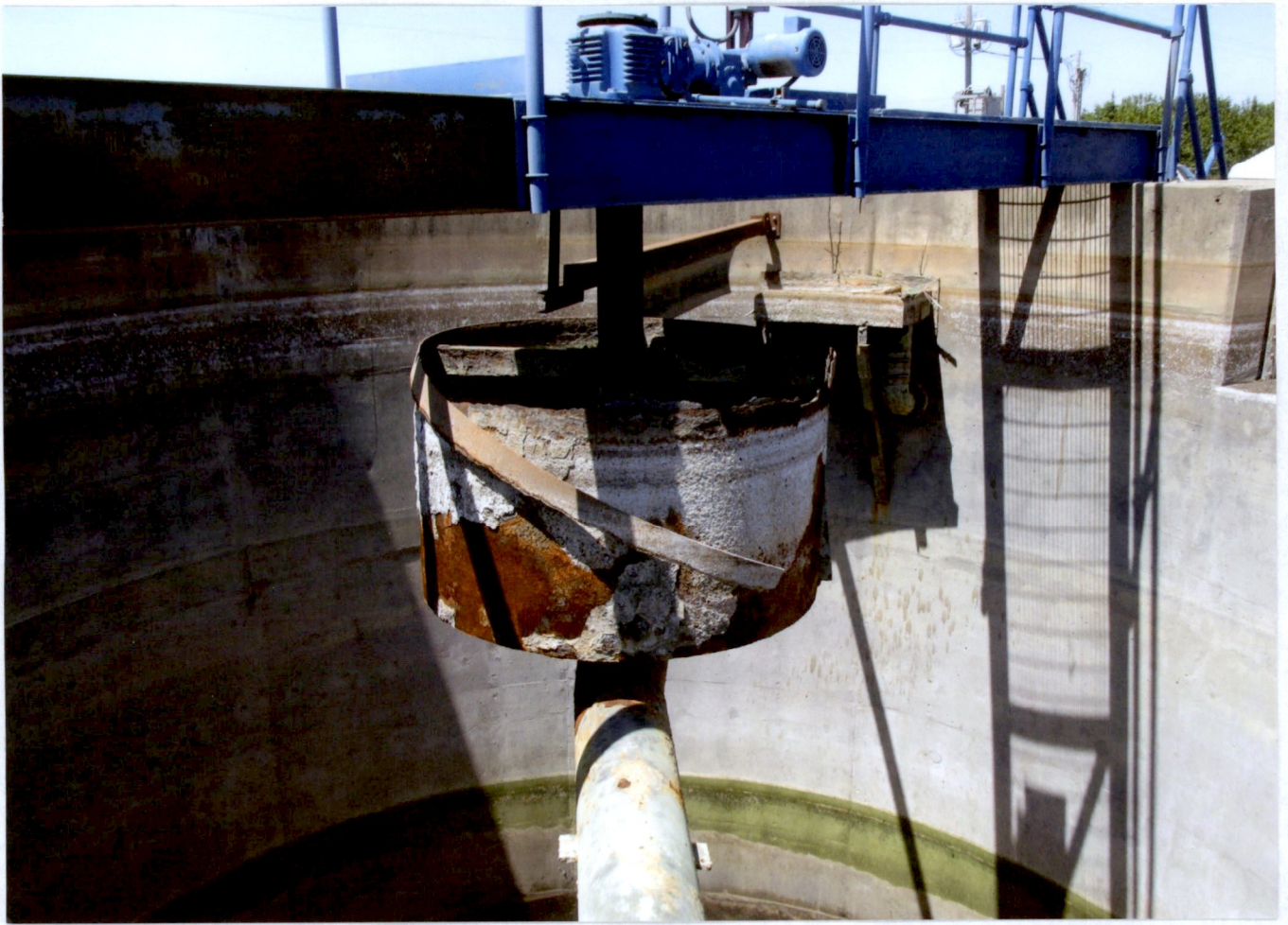
15. WEST SIDE DECANT- DOWN FOR REPAIRS- REPAIRS MADE- BACK IN SERVICE
