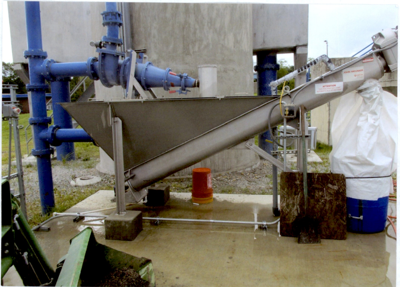
3. METCAN GRIT REMOVAL AND SAND Dewatering SCREW
